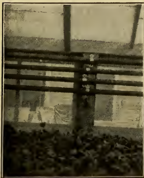
17.—Fastening pipes to posts by tin clips
